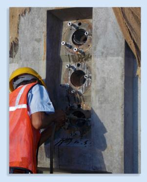
Pressure grouting to prevent active water leakage in water retaining structures, basements and diaphragm walls using
